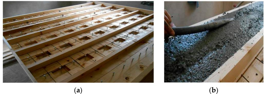
Figure 5. (a) Formwork of TCC beams before casting concrete; (b) Per-vibrator usage.
