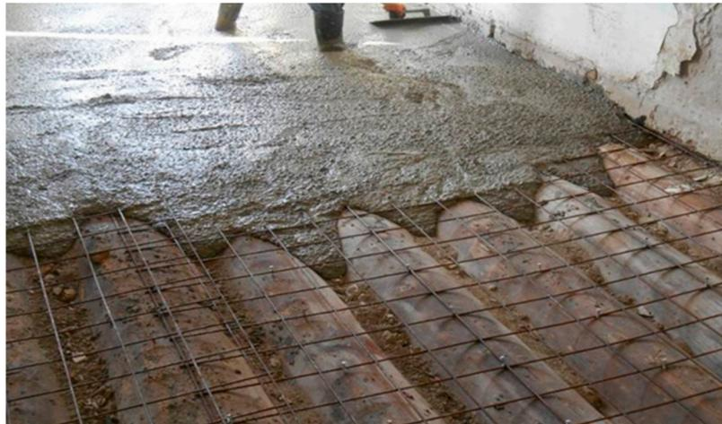
**Figure 1.** Strengthening of the existing timber floor structures of a building with cultural monument status, using the method of coupling with concrete [3].
