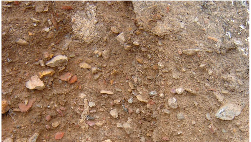
**Figure 5.** Detail of crushed red ceramic and medium-sized stones added to the earth in the rammed-earth Juromenha fortification. Author: M. Rocha, 2022.
