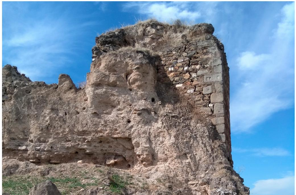
**Figure 10.** Action of water and structural failure in a military rammed-earth structure (Juromenha, Portugal). Author: M. Rocha, 2021.
