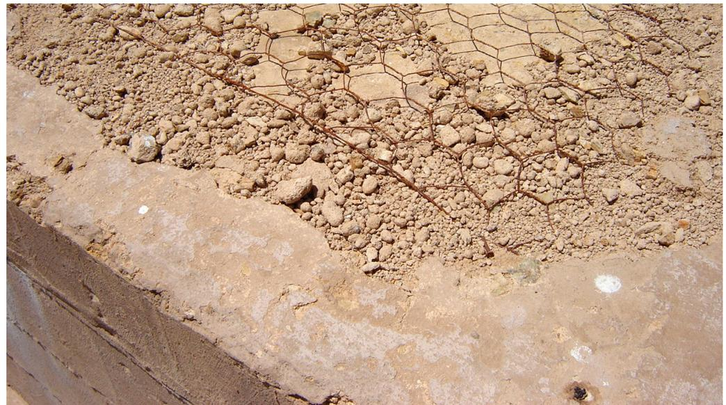
**Figure 12.** Detail of the incompatibility of materials in an intervention for the conservation of a rammed-earth Reina fortification, causing damage to the structure (Author: M. Rocha, 2007).
