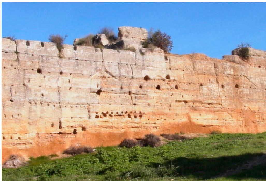
**Figure 3.** Example of a military rammed-earth defensive fortress in Paderne Castle, Portugal; some of the visible holes are from the original formworks used. Author: M. Rocha, 2003.
