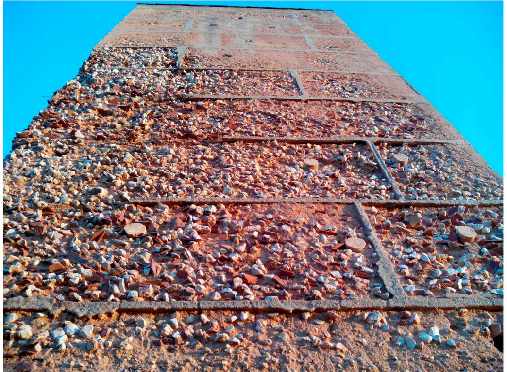
**Figure 13.** Detail of an ineffective intervention for the recovery of volumes in the fortification of Silves, Portugal, simulating rammed earth but distorting the original architectural and constructive concept (Author: M. Rocha, 2016).
