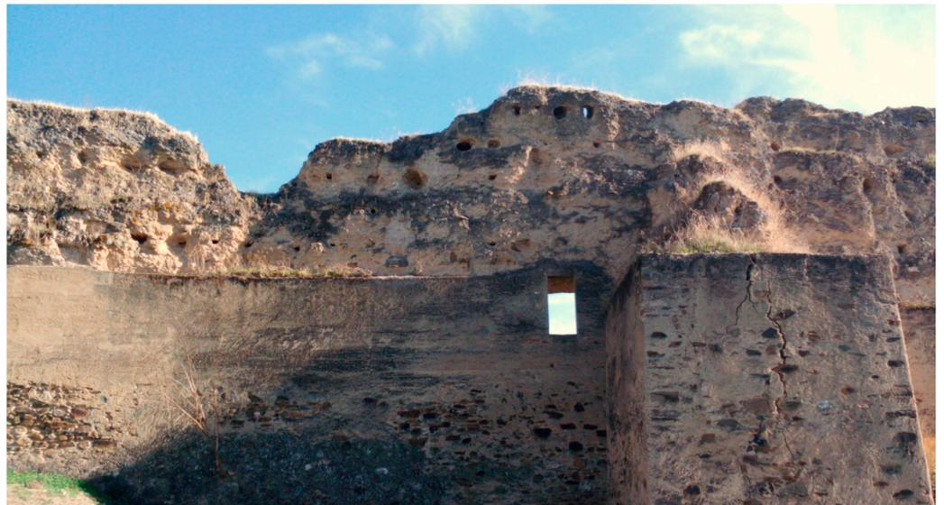
**Figure 14.** Detail of inadequate past intervention for surface repair, with mortar placed inside formworks to simulate rammed earth in the Juromenha fortress, Portugal. Although keeping its integrity for decades, this intervention has a very low visual compatibility (Author: M. Rocha, 2021).
