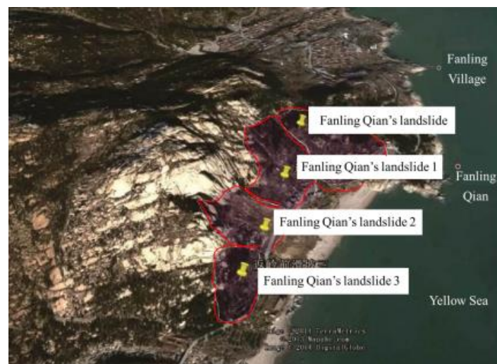
Figure 2. Location map of the Fanlingqian landslide.
