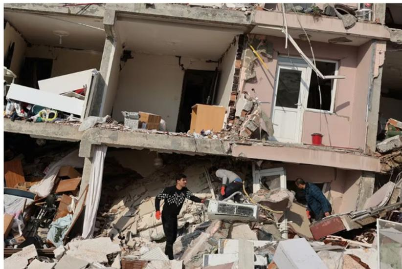
**Figure 3.** Failure to the multilayered infill wall during strong intensity earthquake [22].
