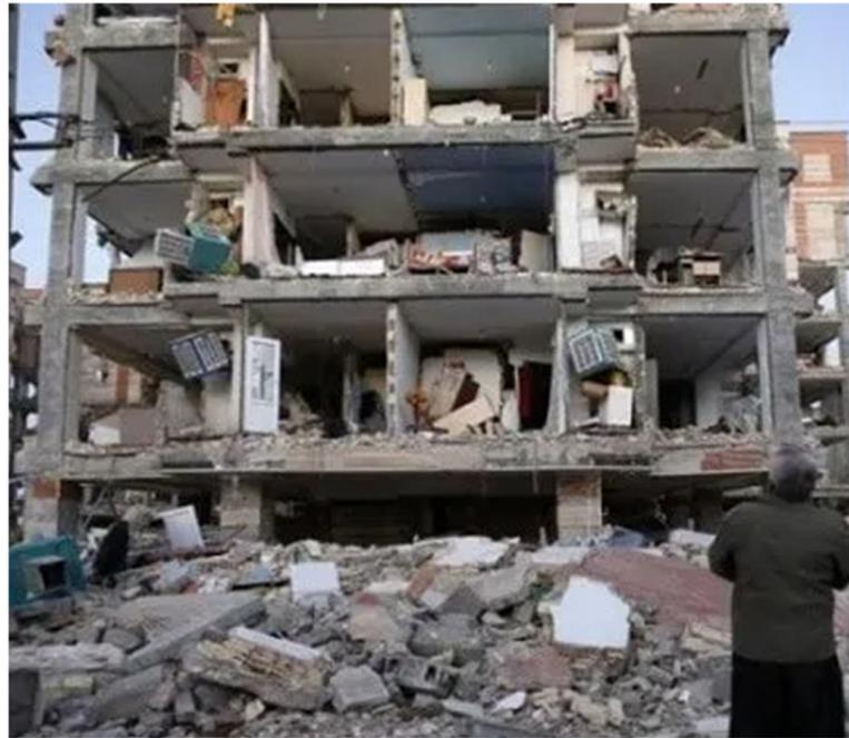
**Figure 2.** Damages to exterior walls in the life safety limit state [37].
