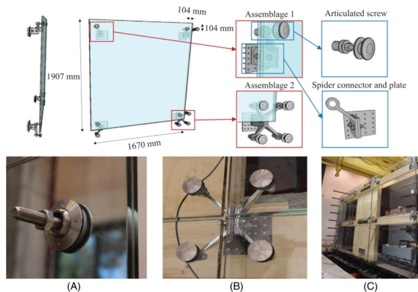
**Figure 8.** (A) Spider ball placed in the glass. (B) Connection of spider. (C) Final wall panel [12].
