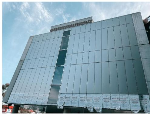
**Figure 1.** Applications of aluminum cladding systems (Belconnen Health Reclad) [2].
