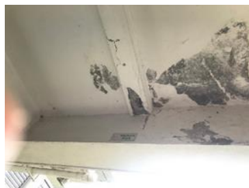
(h) Concrete spalling
