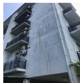
(f) Wall staining due to corroded steel
