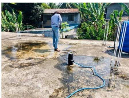
(n) Pressure washing the surface
