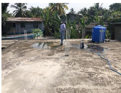
(j) Biological stains on concrete slab
