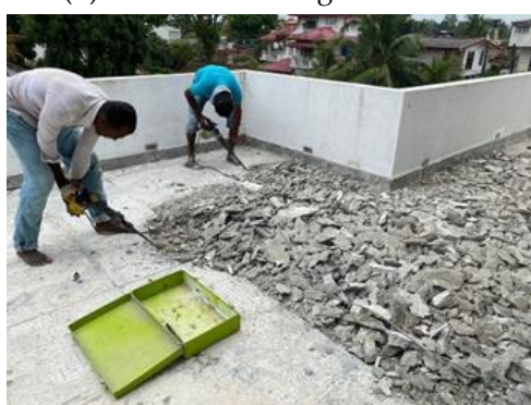
(o) Jackhammering the surface
