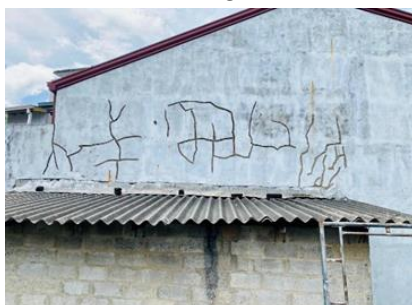
(l) Enlarged cracks to apply seal.
