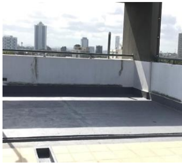
(c) Parapet wall crack
