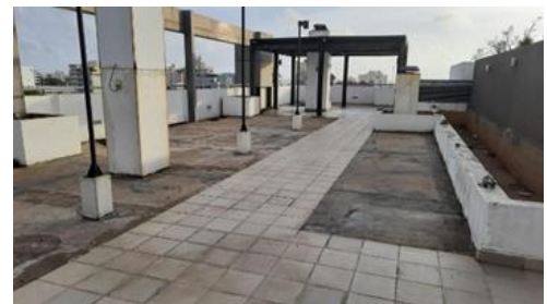
(e) Removing the top layer of the surface.
