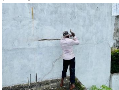
(k) Routing cracks
