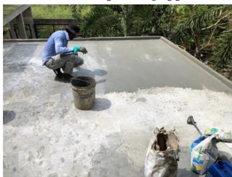
(q) Applying a waterproofing layer
