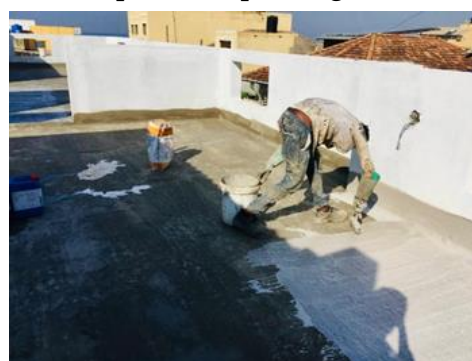
(q) Applying a waterproofing layer
