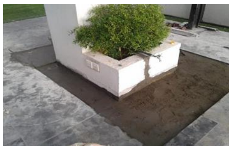
(f) Leveling substrate using mortar
