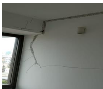
(j) Wall crack
