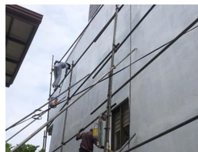
(m) Finishing wall after repairing cracks.
