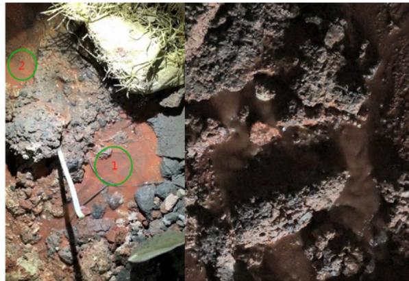
**Figure 11.** Seepage of groundwater from the inverted arch near K4 + 914.
