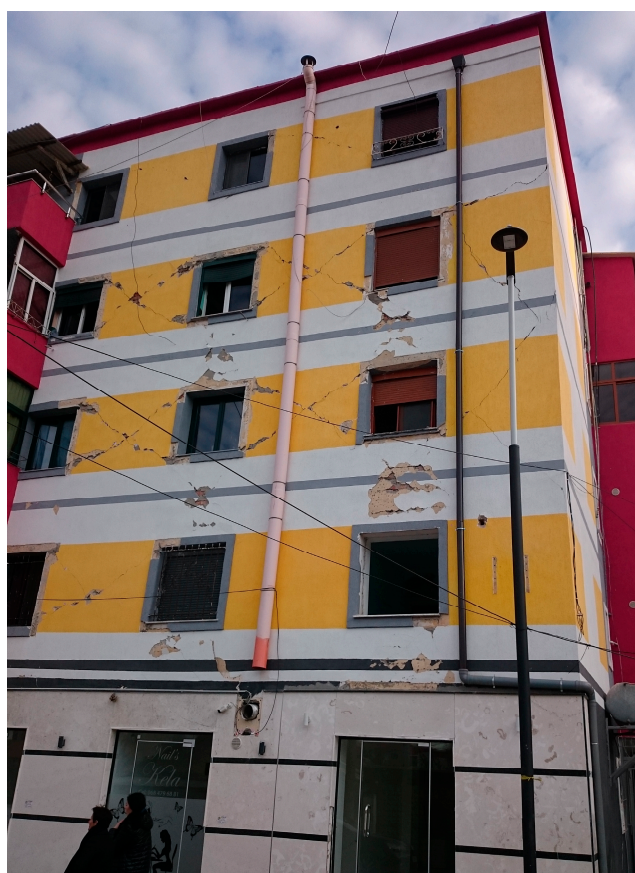
Figure 14. Shear cracks stemming from diagonal tension in residential masonry buildings in Albania.
