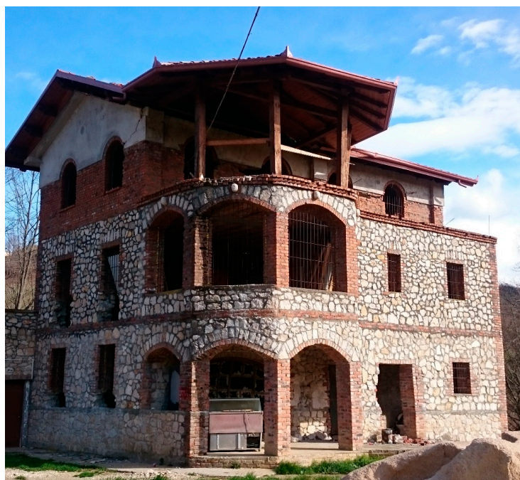
Figure 10. Masonry dwelling with large openings and wooden lintels above openings in Vore. The 1st and 2nd floors are constructed of stone brick while the 3rd story is built of clay bricks.
