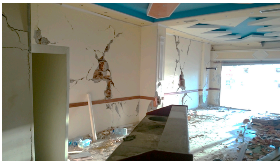
Figure 4. Infill wall damage in an RC building due to out-of-plane bending and shear failure.
