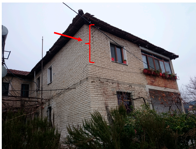
Figure 13. Separation of walls because of improper connection between the roof and the underlying masonry and flexible top floor.
