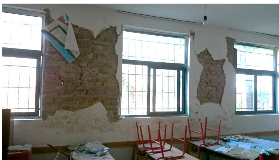
Figure 5. In-plane shear failure of inadequately confined masonry wall due to windows opening.
