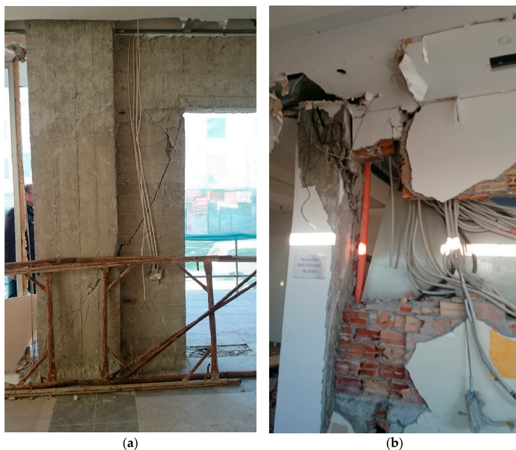
Figure 6. Shear failure of columns on RC buildings in Durrës. (a) Typical shear failure of columns; (b) Buckling of rebars in plastic hinge regions of columns due to insufficient transverse reinforcement.
