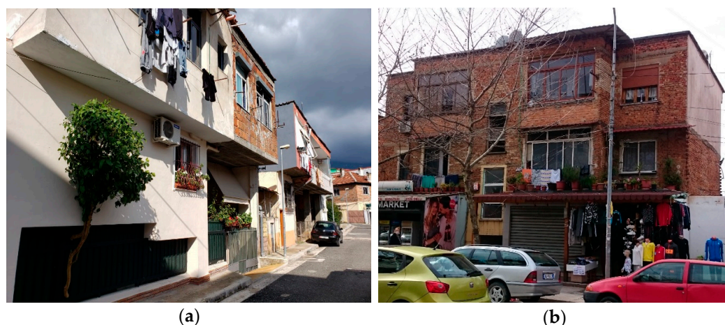
Figure 11. Intervention examples on URM buildings: (a) expanded overhangs as balconies and use of different construction materials; (b) Interventions done after its construction on the ground floor (New openings).
