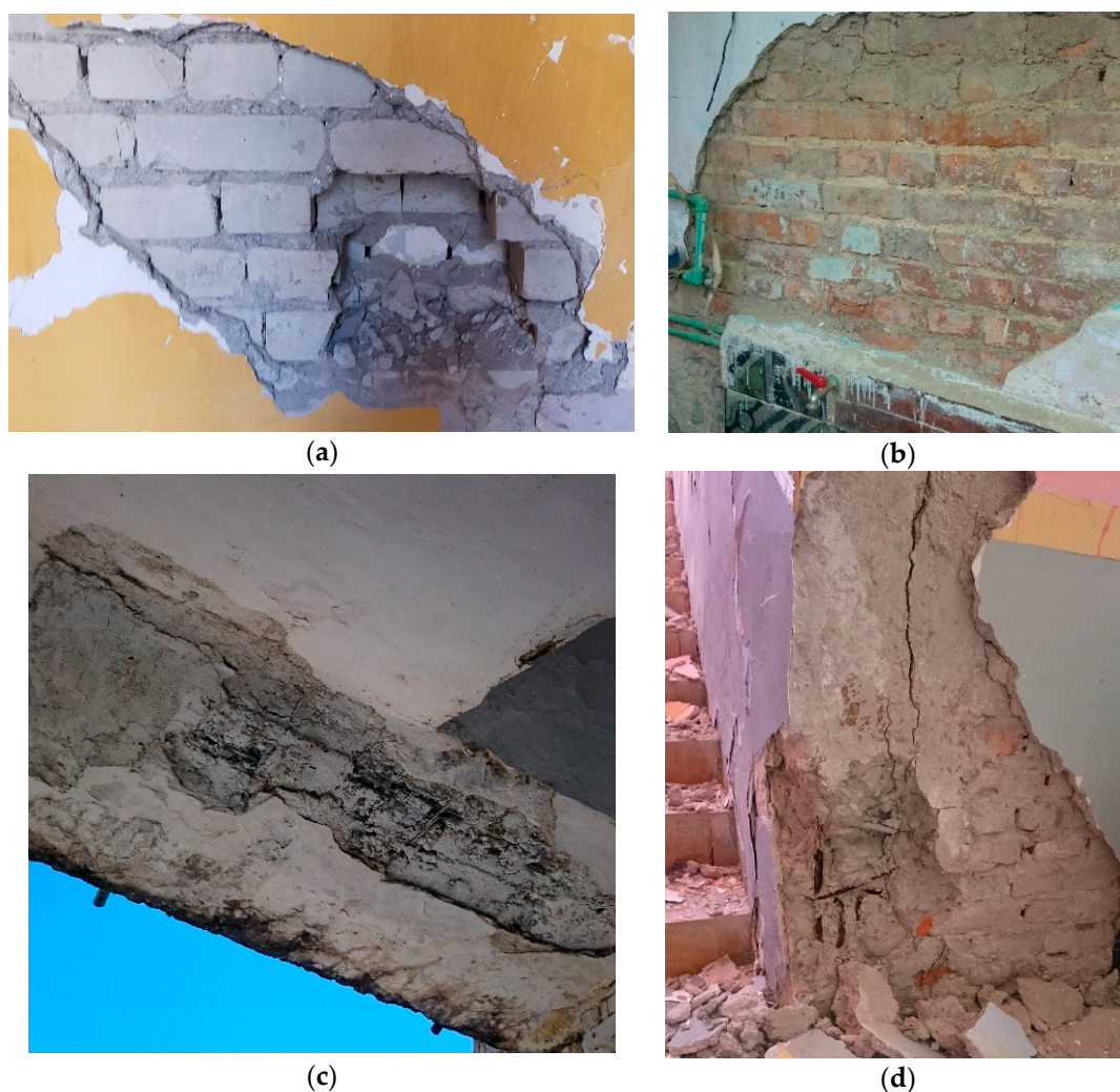
Figure 9. Typical solid bricks and details of the confinement elements used for masonry walls: (a) Silicate bricks; (b) Red clay bricks; (c,d) RC beams and column reinforcements.
