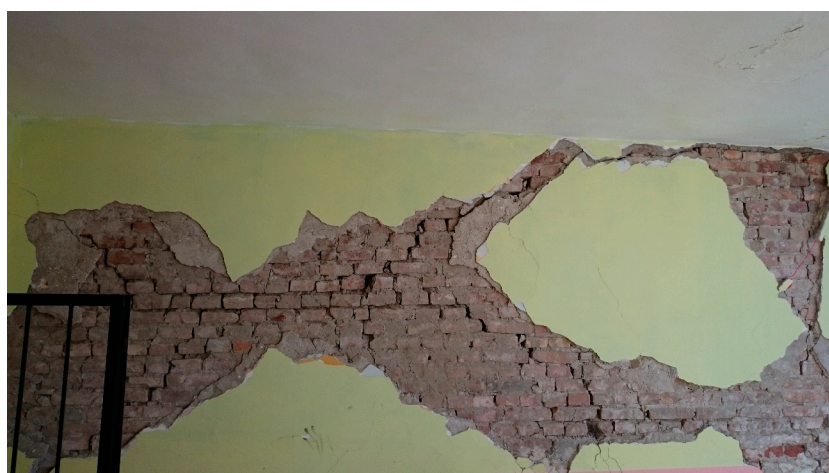
Figure 18. Showing shear cracks and in-plane failure of the masonry walls.
