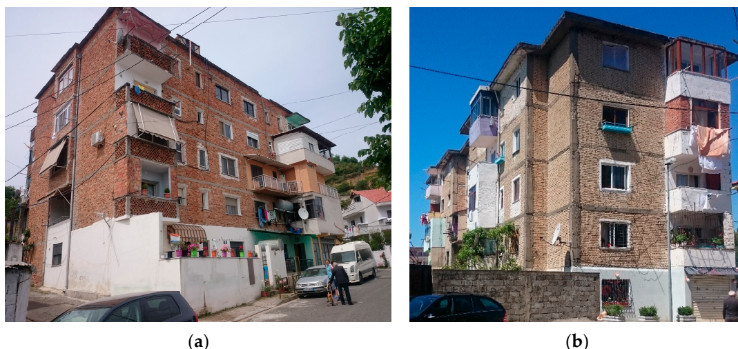
Figure 8. Typical masonry buildings (a) URM; (b) Confined masonry.
