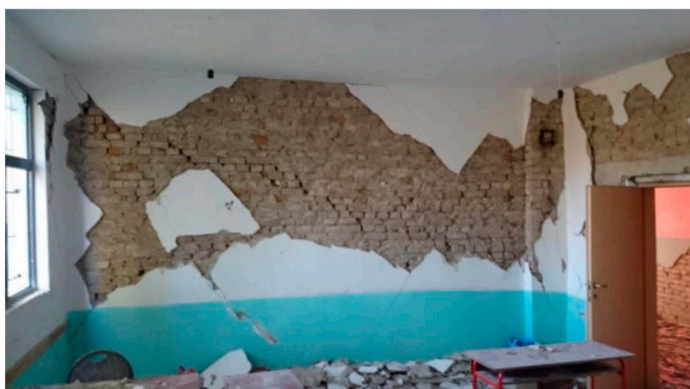
Figure 19. Damage pattern observed on load-bearing wall of the masonry school building.
