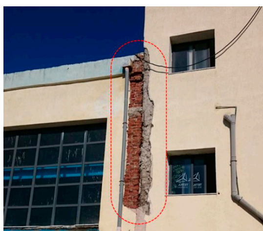
Figure 15. Pounding failure b/w adjacent masonry and RC buildings.
