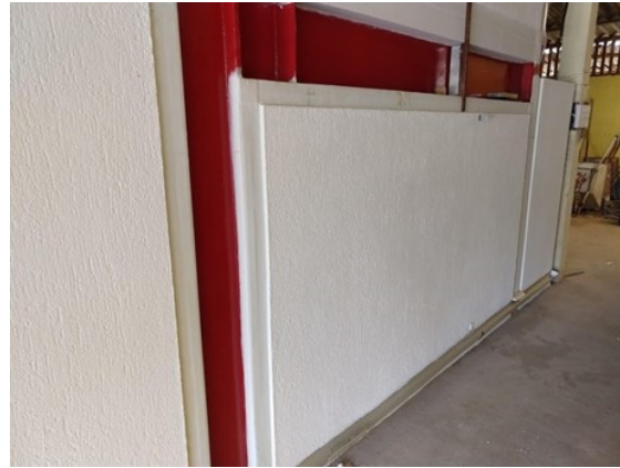
Figure 13. General appearance of the wall after its external surface was painted.
