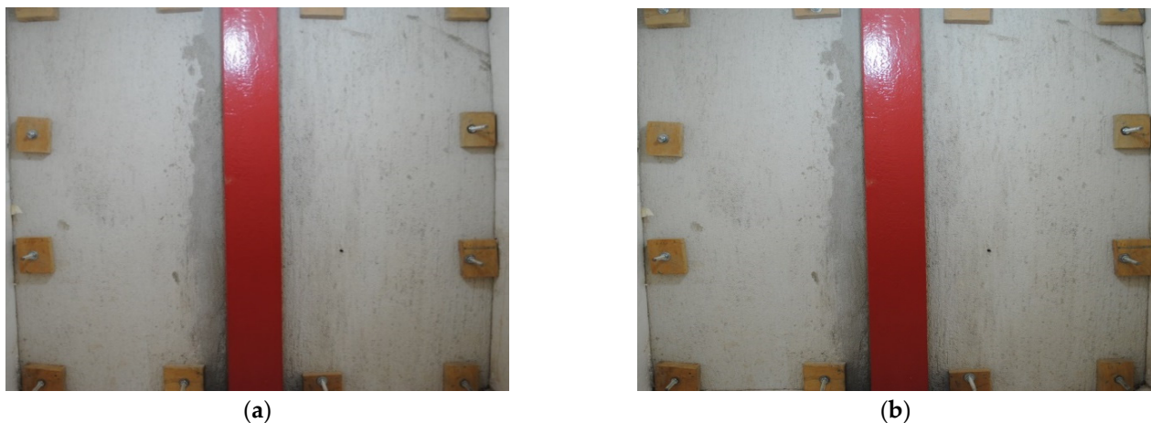
Figure 25. Appearance of the INT1 specimen's inner face before and after the watertightness test: (a) before; (b) after.
