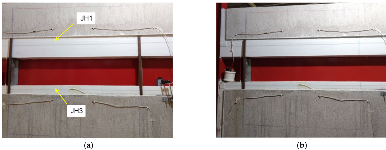
Figure 19. Appearance of interface INT2 in specimen E2: (a) before the heat exposure and thermal shock test; (b) after the test.
