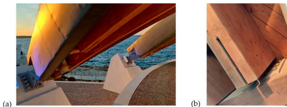
**Figure 1.** Joints of timber structural members: (a) pinned joint, (b) moment joint.
