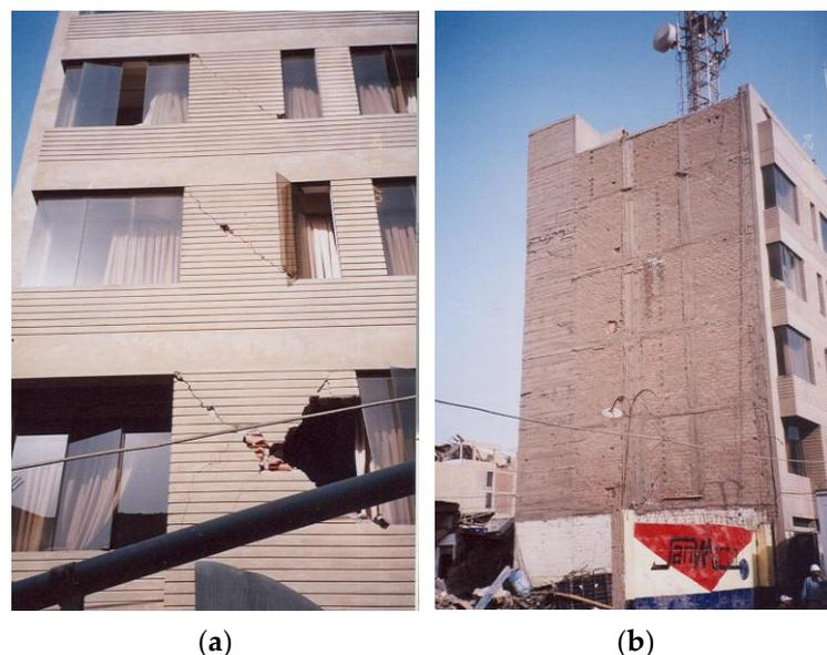
**Figure 28.** Damage sustained by the Candelabro Hotel building in the 2007 Pisco, Peru earthquake (M 8.0): (a) damage to masonry piers, showing the absence of vertical RC confining elements in longitudinal wall; and (b) undamaged solid CM walls in the transverse wall (photos: D. Quiun).
