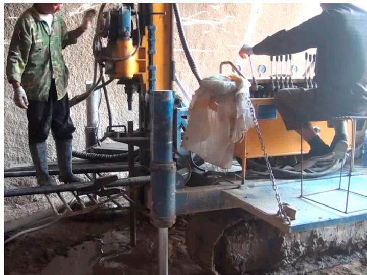
**Figure 3.** On-site construction diagram of the tunnel-based jet grouting pile.
