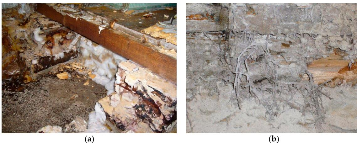
**Figure 4.** Photograph of wood-decay fungus sporocarp on wooden element (a) and visible root system of wood-decay fungus (b).
