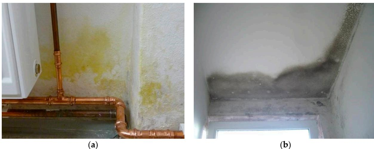
**Figure 6.** Example of real occurrence of moulds (microscopic fungi): (a) on masonry; and (b) ceiling structure surfaces.
