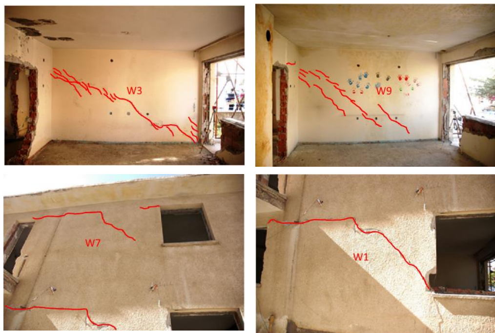
Figure 6. Damage distributions of the tested two-story masonry building (from [101]).
