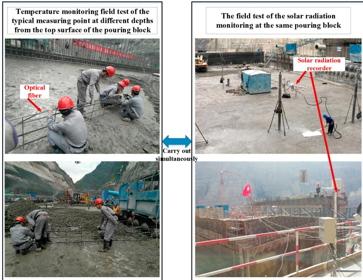
**Figure 6.** Diagram of the temperature and solar radiant monitoring field test.
