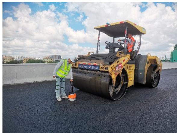
**Figure 7.** SMA-13 compaction test with different numbers of rolling times.
