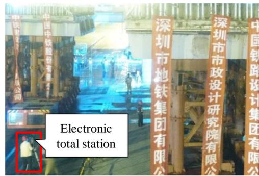
Figure 12. The electronic total station used in the site.
