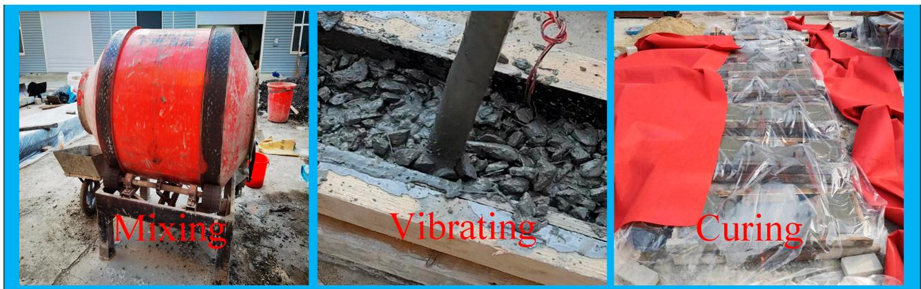
Figure 3. The specimen fabrication process.
