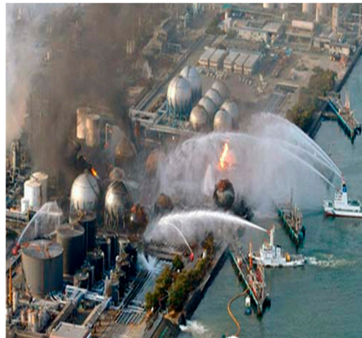
Figure 1. Fukushima nuclear leakage accident in Japan.
