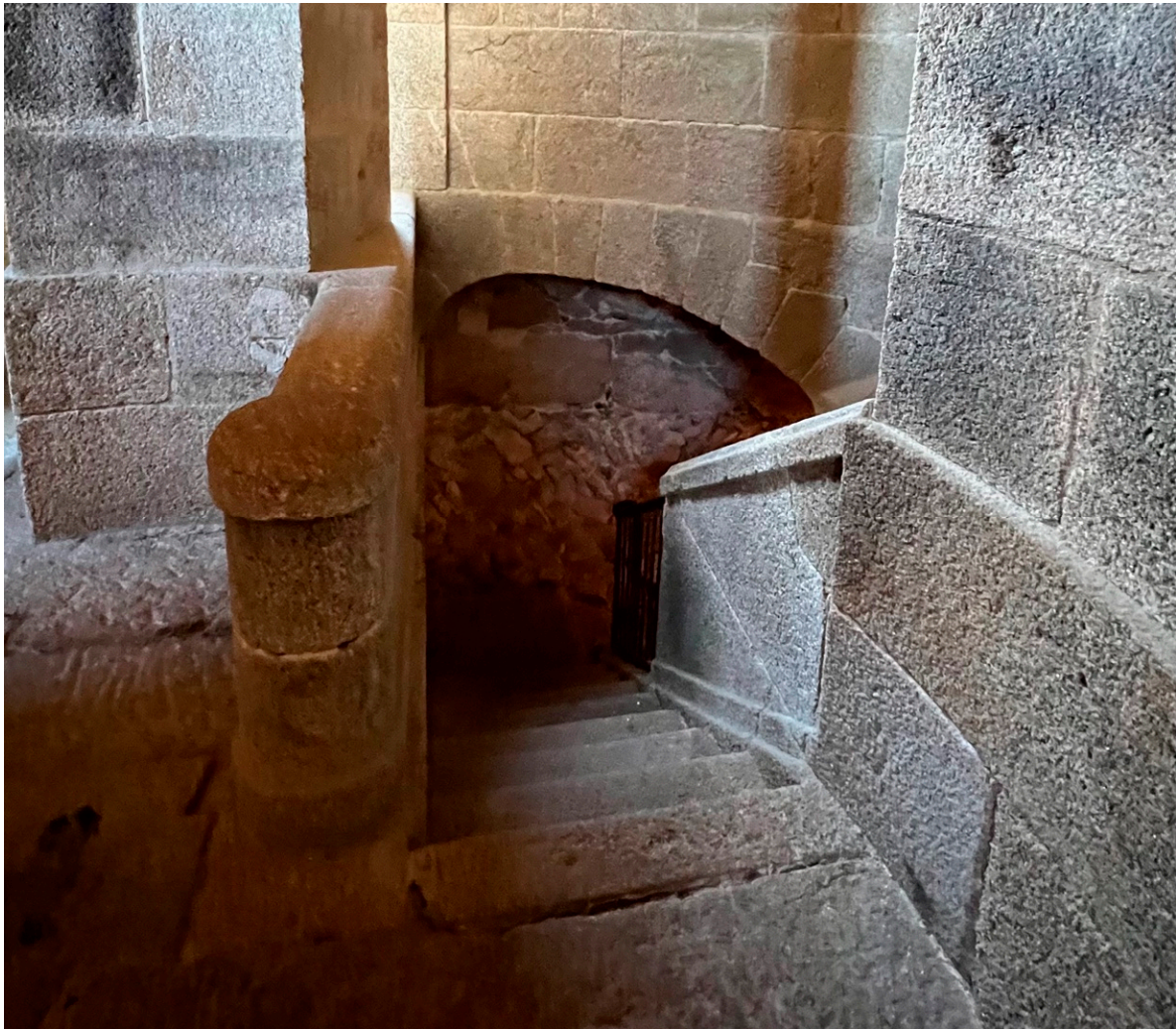
Figure 12. Arrival of the stairs at the level of the Eustaquio Giannini roundabout.
