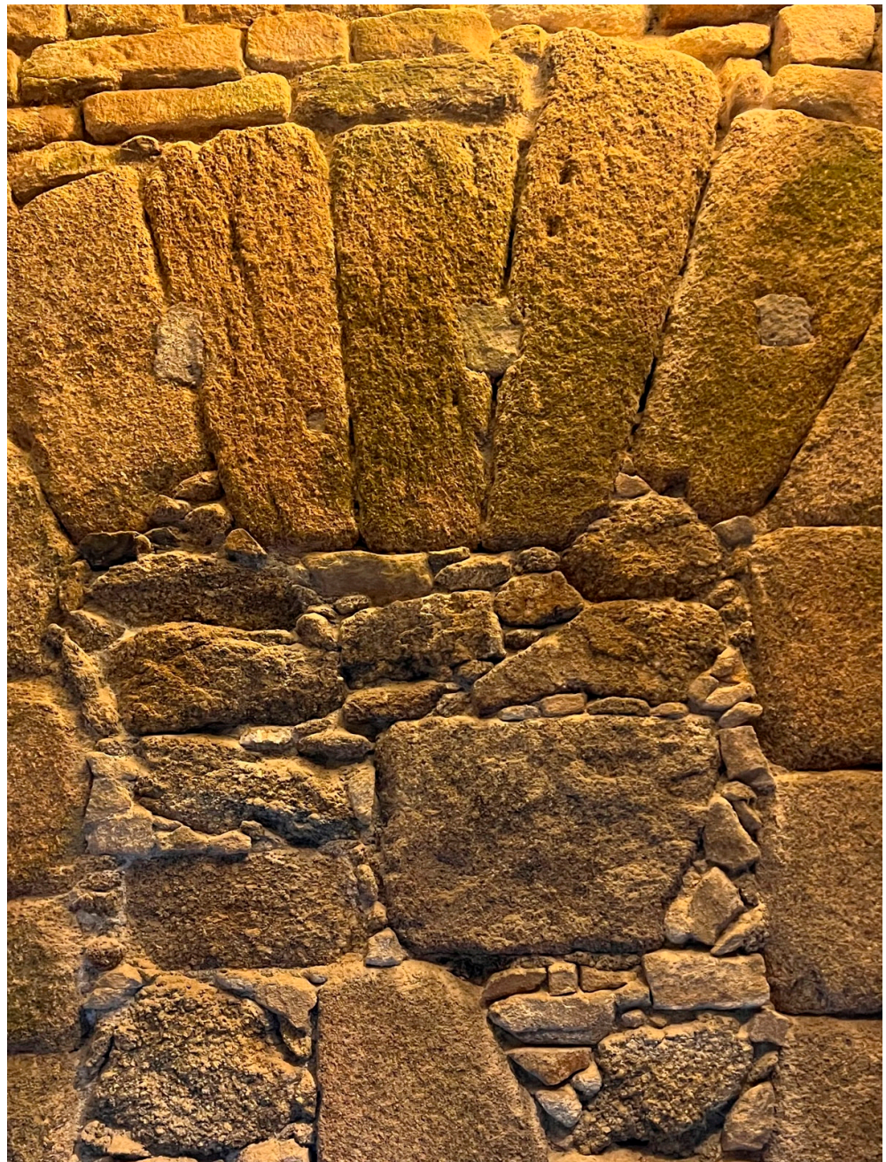
Figure 16. Inner chamber. Closed opening detail, with jambs and voussoirs much larger than the masonry of the wall.
