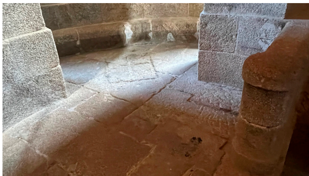
Figure 17. Flooring of the upper rotunda with the double T slabs that tie the structure together.
