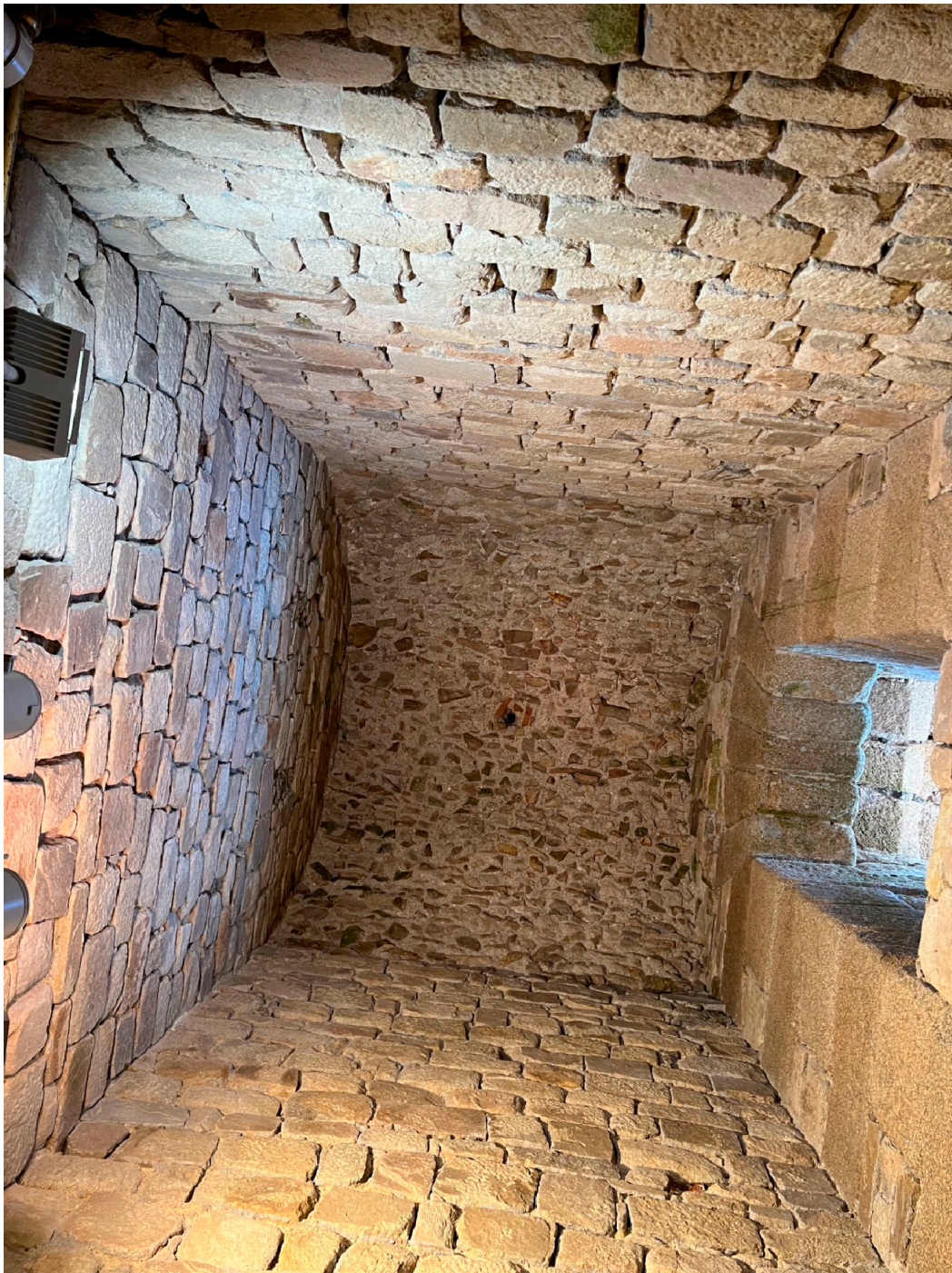
Figure 15. Barrel vault of one of the chambers, showing the placement of the stones and their size in relation to the masonry of the walls.
