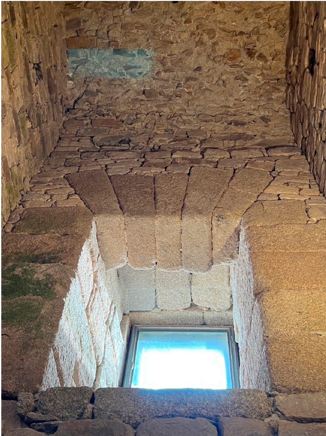
Figure 14. Inner chamber. One of the windows of the current stairwell. The larger stones were used in the formation of holes, the smaller ones in the walls and the smaller ones in the vaults.
