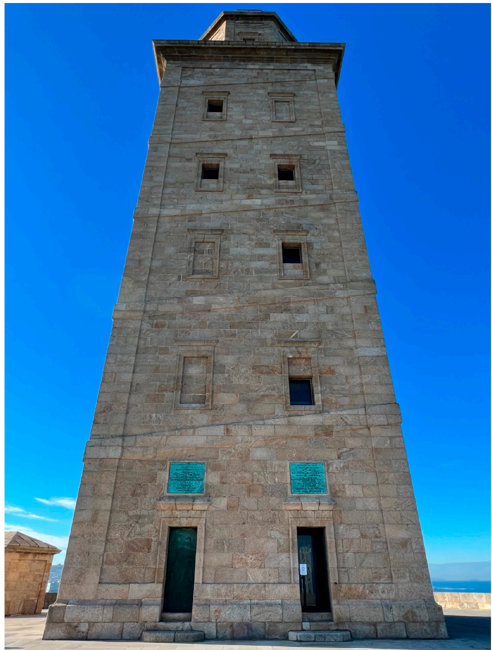
Figure 9. Main façade (northeast orientation) of the Tower of Hercules, where you can see the access doors, on which two bronze plates were placed commemorating Giannini's restoration.
