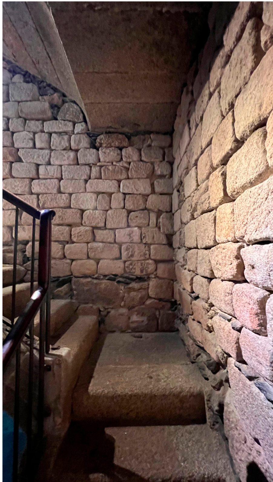
Figure 8. View of a section of the stairs installed by Giannini, where you can see the black stones that facilitated the fixing of the stairs on the Roman masonry.
