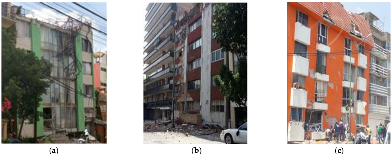
Figure 1. Examples of upper soft-story failures in Mexico City caused by the 2017 Mw7.1 Morelos–Puebla seismic event. (a) 241 Rebsamen St., Narvarte neighborhood; (b) 37 Patricio Sanz St., Del Valle Norte neighborhood; and (c) 47 Gallinas St., Lomas Estrella neighborhood.
