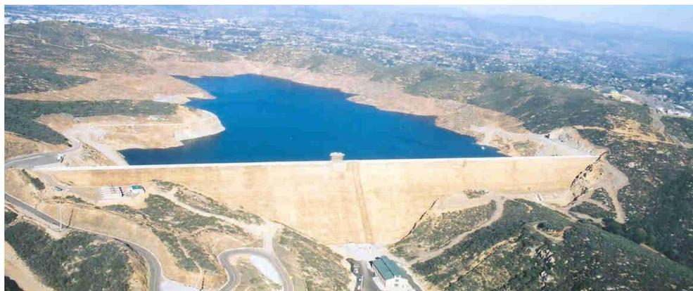
Figure 1. Roller-compacted concrete dam Olivenhain, USA, 2004.
