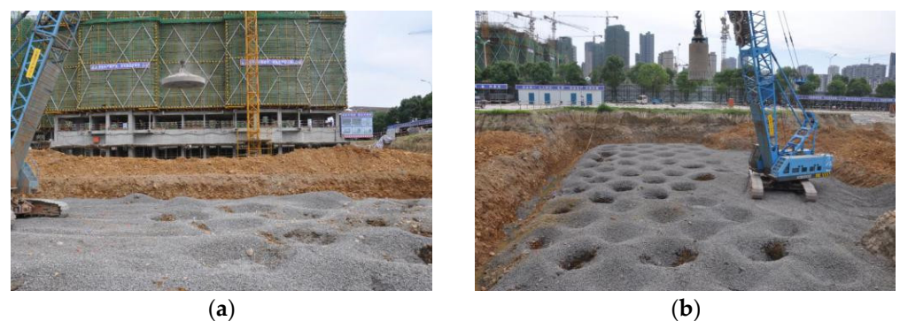
Figure 4. Construction photo of combined hammer: (a) flat hammer; and (b) column hammer.
