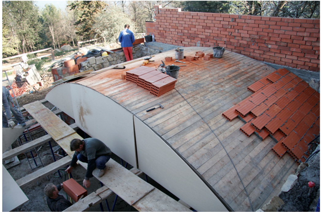
Figure 5. Contemporary process of execution of a tile vault.
