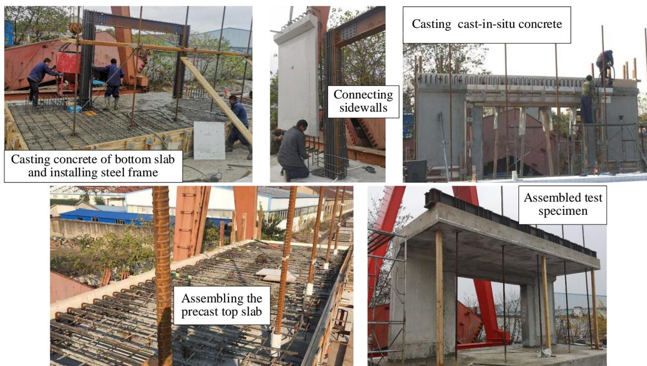
Figure 5. Construction process of the test specimen.
