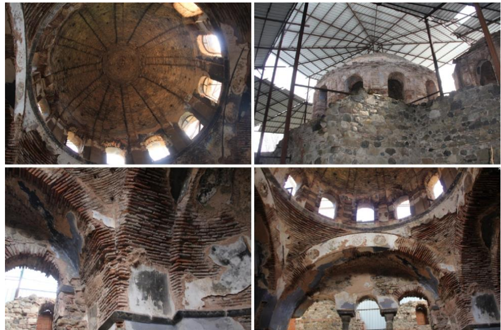
Figure 5. Views of domes, arches and pendentives at naos.
