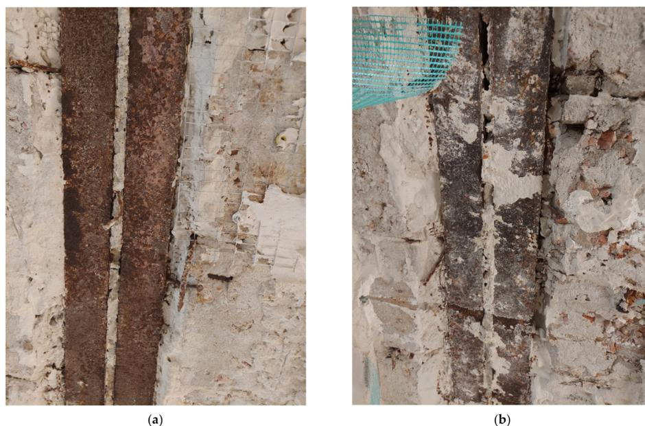
**Figure 5.** Technical condition of the bottom chord of the steel trusses: general view of the bottom chord of the steel trusses in different places (a) the finishing layer had no adhesion to the surface of the bottom chord; (b) the finishing layer had good adhesion to the surface of the bottom chord.
