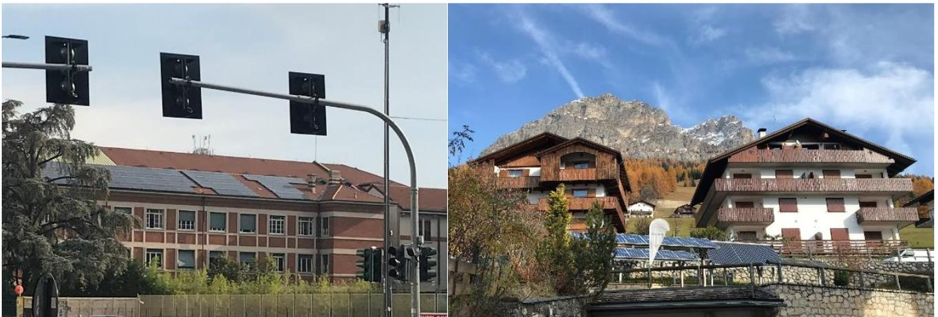
**Figure 9.** Negative examples of the “*recognizability*” criteria of the solar intervention in a XX Century School in Milan (Italy) and in traditional alpine buildings in Val Sarentino (Italy) where PV and ST panels are visible from public spaces for their irregular shapes, blue colors, and high reflectance (Source: Elena Lucchi).
