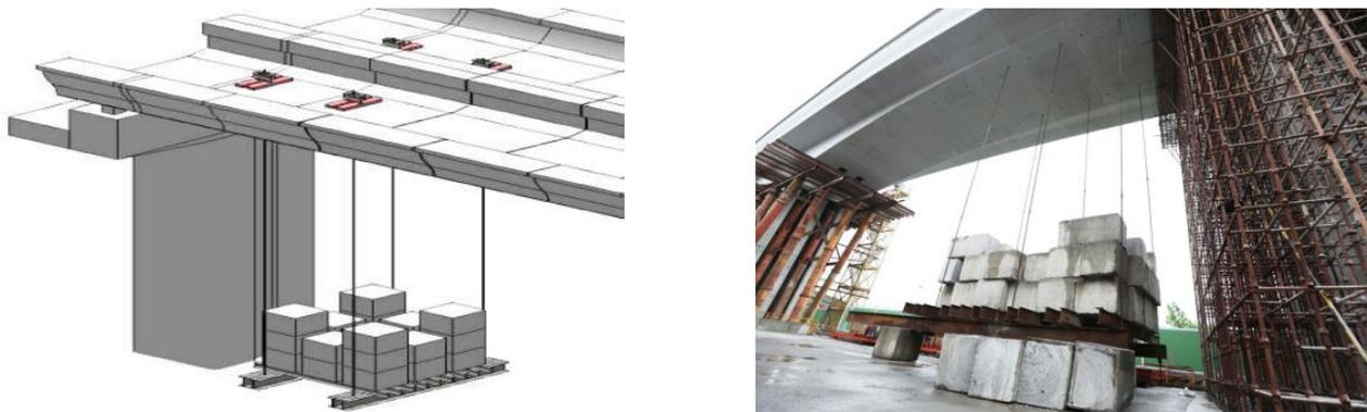
**Figure 8.** Side-span counterweight.
