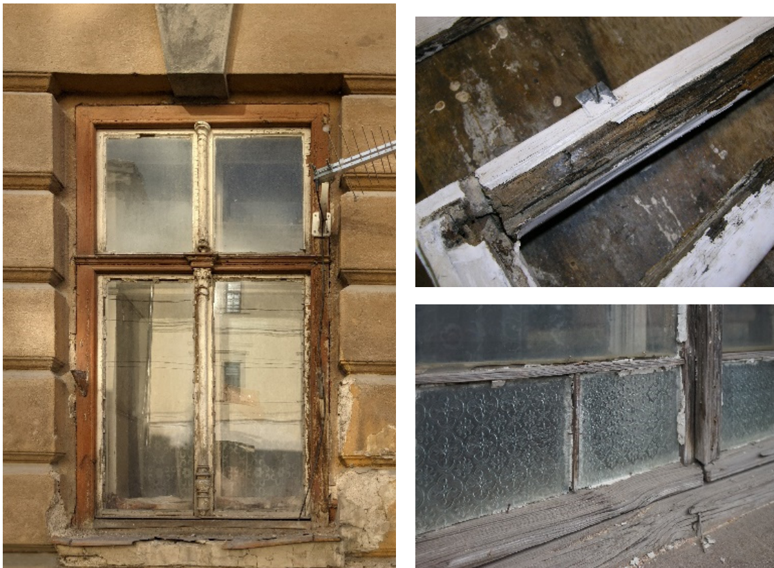
Figure 1. Examples of windowpanes in urban tenement buildings with neglected maintenance, mainly showing failures caused by cyclical changes in atmospheric influences (Photographs by K. Kroftova).
