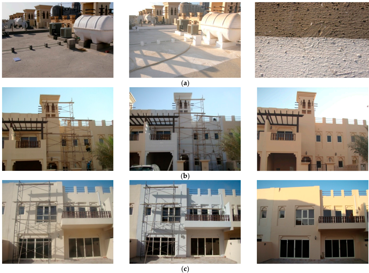
Figure 7. Picture showing retrofitting townhouse with cool roof and cool walls. (a) Roof coating: before (left) and after (middle); with and without SRI paint right). (b) Wall coating, front facade: before (left), after primer coating (middle) and after both top coatings (right). (c) Walls coating back facade: before (left), after primer coating (middle), and after both top coatings (right).
