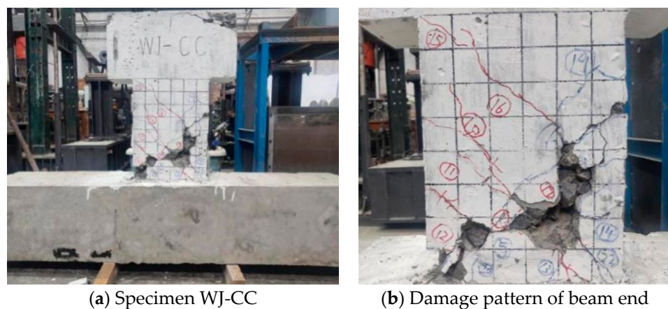
Figure 5. Failure condition of specimen WJ-CC.
