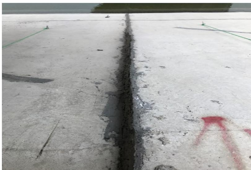
**Figure 2.** Typical cracking and settlement of a channel lining panel.
