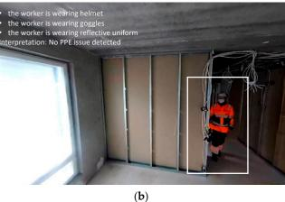
**Figure 2.** The same image but different interpretations based on different goals. (a) Interpretation of the operation progress states represented in the image; (b) interpretation of checking the worker is wearing personal protection equipment (PPE) appropriately.
