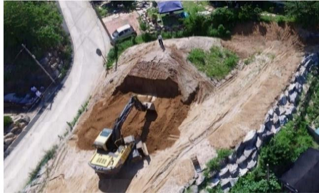
**Figure 3.** Slope cutting mechanism using excavator.
