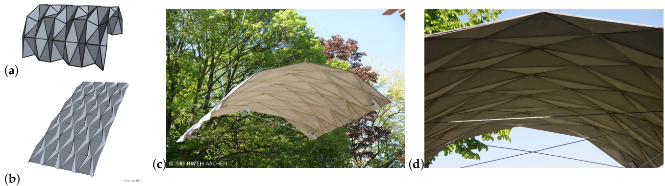
Figure 1. (a,b) Waterbomb folding structure: different choices of folding angles of the base cell lead to different curvature of the whole waterbomb structure; (c,d) Photograph of a carbon-reinforced concrete roof prototype folded using origami tessellation kinematics (Photographs: Rostislav Chudoba).
