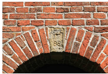
Figure 3. A stone arc is stable only when all stones are included (Photograph: Franz Vincentz [20]).
