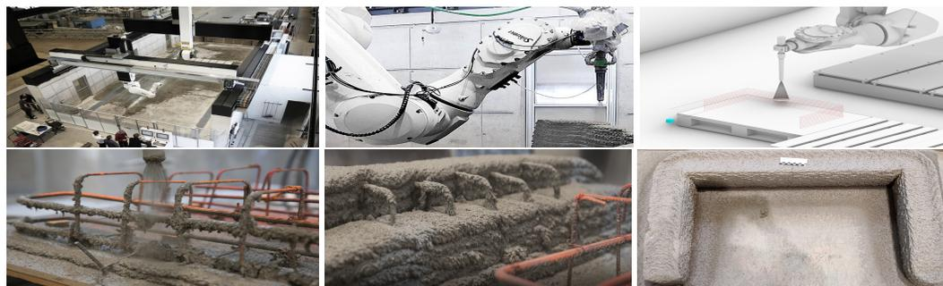
**Figure 21.** Robotic printing process for construction of the U-shape frame (DBFL, ITE and TU-Braunschweig).
