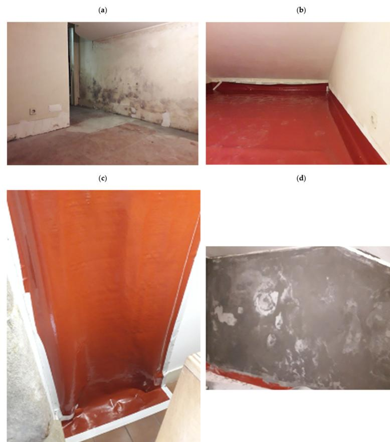
**Figure 4.** A sequence of works carried out. (a) Initial appearance before the execution of the tasks; (b) barrier membrane application; (c) sealing of the outer compartment door; (d) application of mortar to the compartment walls.
