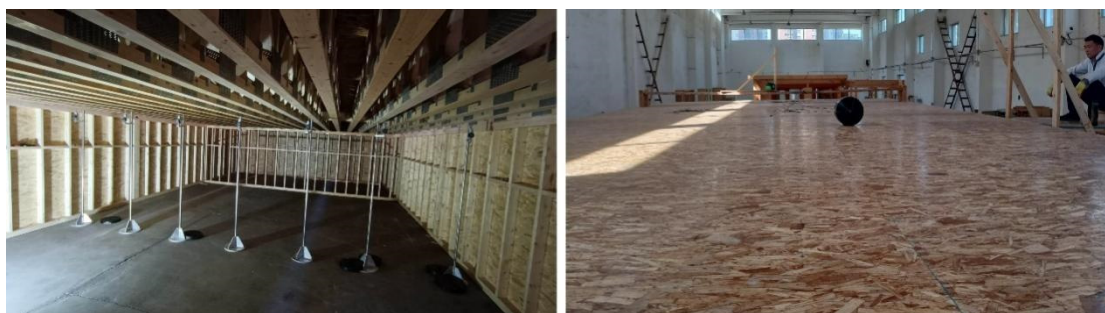
Figure 9. 1 kN static load deflection test.
