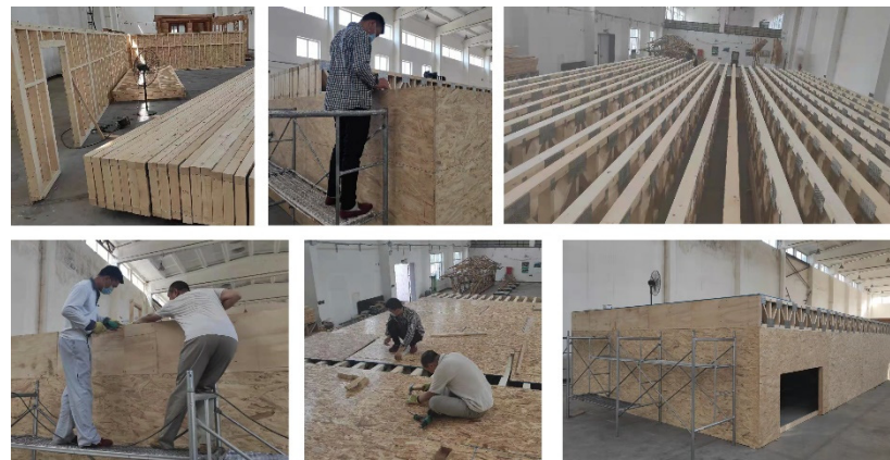
Figure 1. Construction of test floor.
