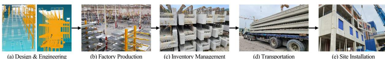
**Figure 2.** Supply chain in OSC production method.
