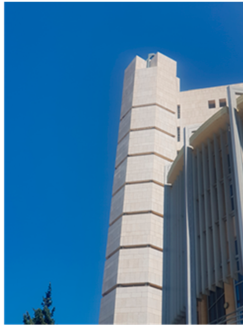
Figure 10. Exterior envelope (Maintenance Indicator = 2.5).
