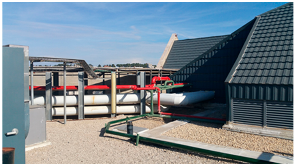
Figure 11. Roofing and installations (Maintenance Indicator = 2.5).
