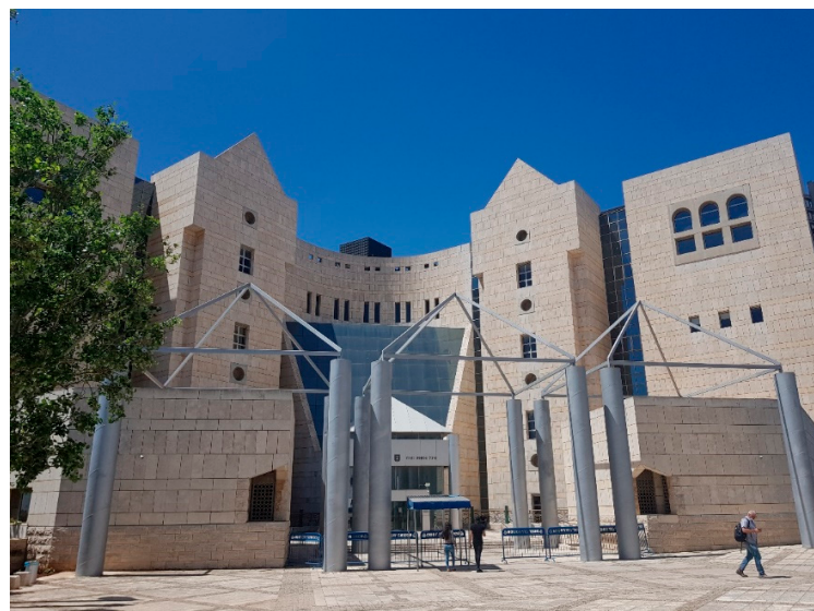
Figure 9. Overview of the building.
