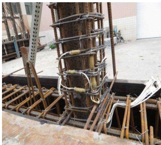
Figure 2. The construction details of an SRUHSC frame.
