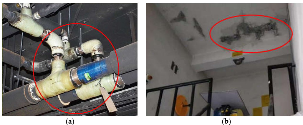
Figure 1. Common forms of damage to ACWS pipe networks: (a) leakage causes ACWS performance degradation; (b) ACWS water leakage causes mildew.
