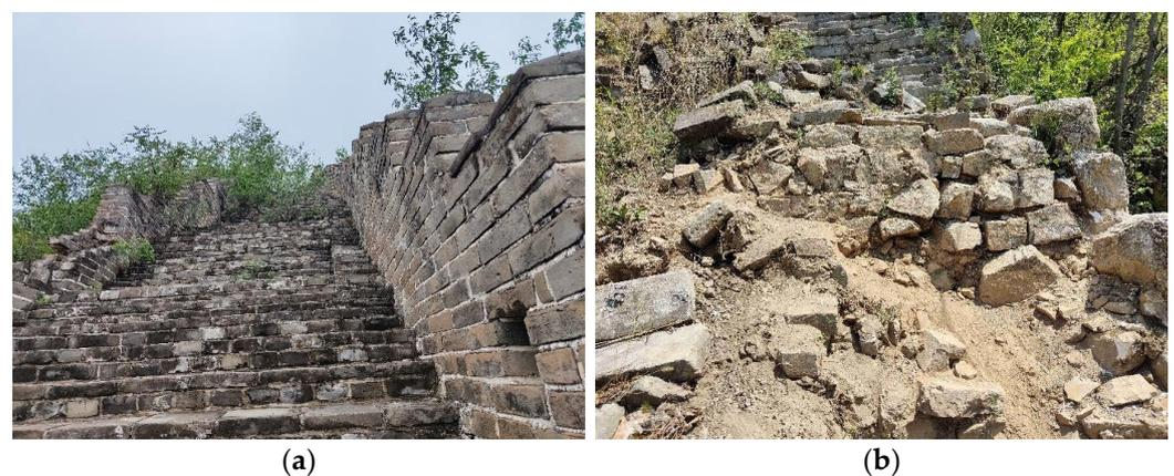
**Figure 7.** Slope section of the great wall: (a) Normal; (b) Collapsed steps.
