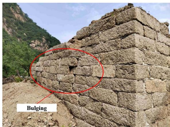
Figure 9. Bulging base wall.
