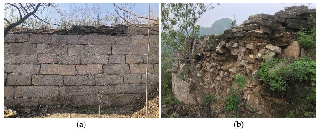
**Figure 6.** Flat section of the Great Wall: (a) Normal stone layer of the base wall; (b) Stone layer collapse.
