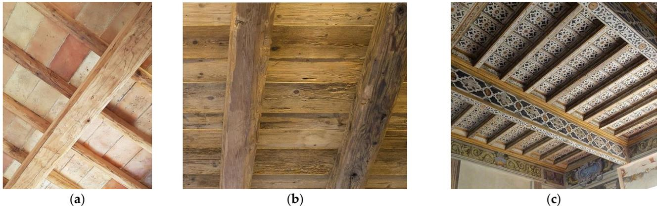
**Figure 1.** (a) Tiles, rafters, and beams; (b) timber beams and boards; (c) decorated timber beam floor: tiles, and two layers of rafters and beams.
