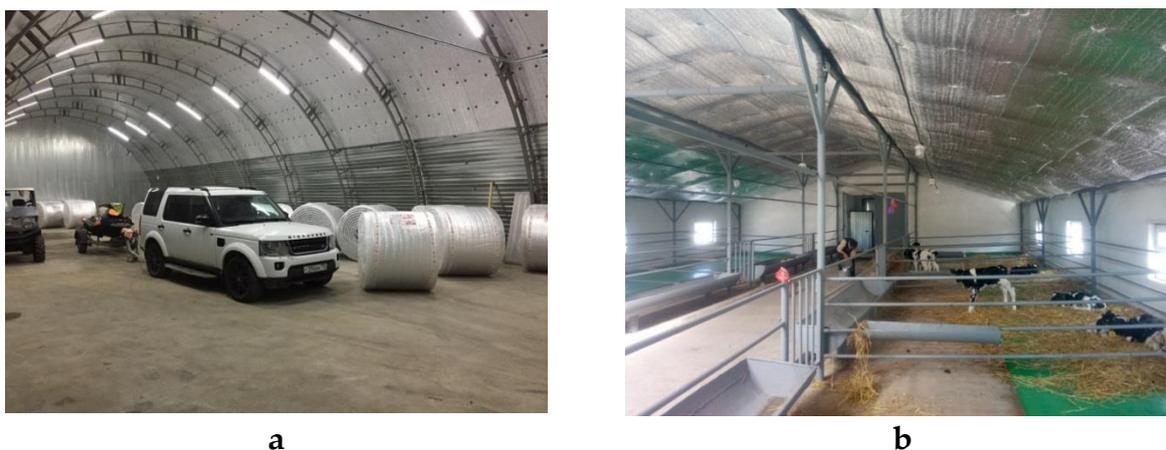
**Figure 11.** Insulation of technological objects: (a)—insulation of parking lot (frameless building); (b)—covered cattle yard (framed building).
