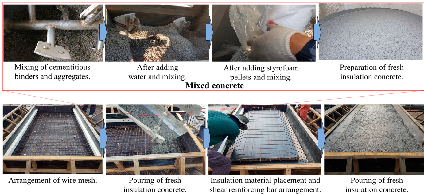
Figure 4. Casting of concrete in the insulation-panel specimens.
