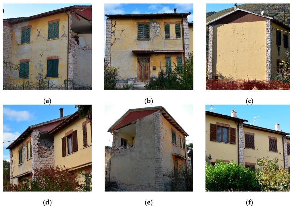
**Figure 8.** Details of damage pattern in IACP building: diagonal shear cracks of piers in (a) north and (b) south facades of unit no. 6, and activation of overturning in west facade; (c) shear cracks in east facade of unit no. 1; crumbling and overturning in (d) east and (e) west facades of unit no. 6; (f) sliding cracks at floor level in unit no. 4.
