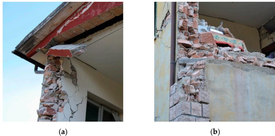
**Figure 6.** Details of unreinforced ring beams at (a) ceiling and (b) floor levels.
