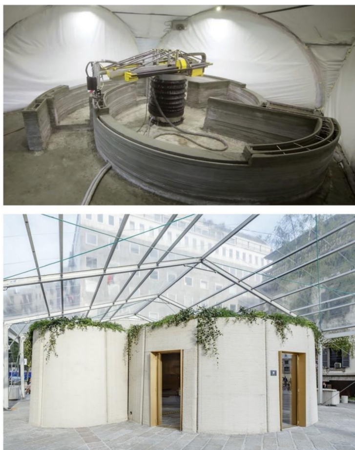
Figure 1. Examples of printed constructions by companies Apis-Cor, reprinted from [4], and Cybe, reprinted from [5]. The pictures show the printing process of a house and an exhibition prototype built in Milan, Italy.
