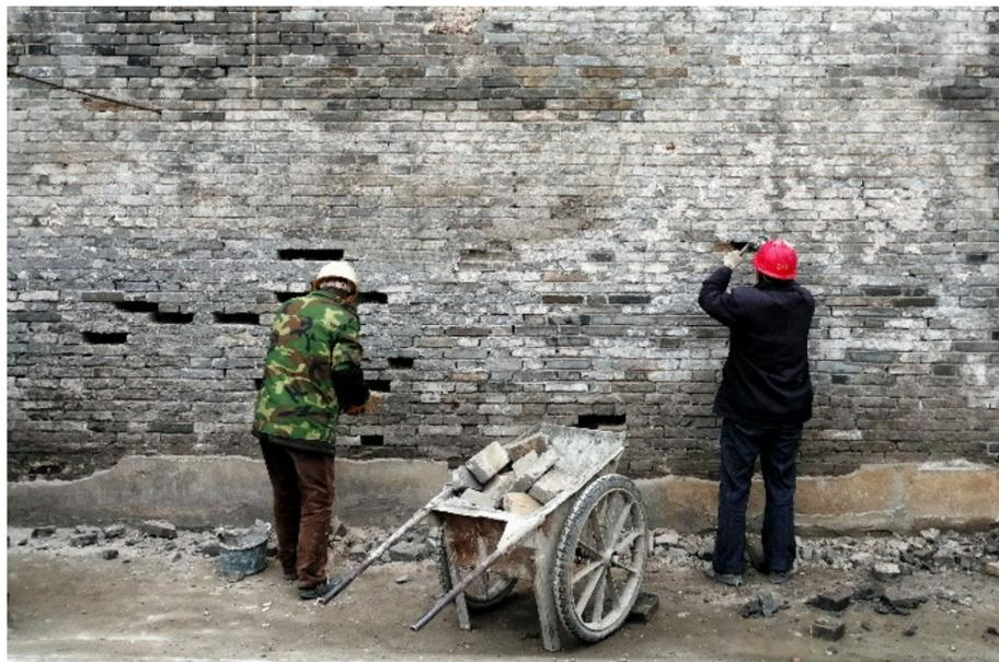
**Figure 22.** Restore the exterior walls with different methods according to the damage degree of the bricks.
