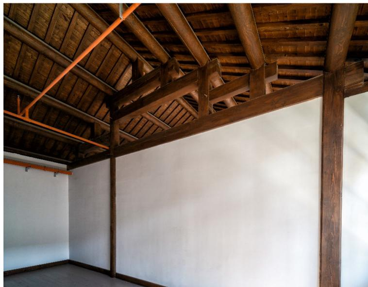
**Figure 19.** The traditional Chinese roof-truss system of “Tianbaoli” townhouses.
