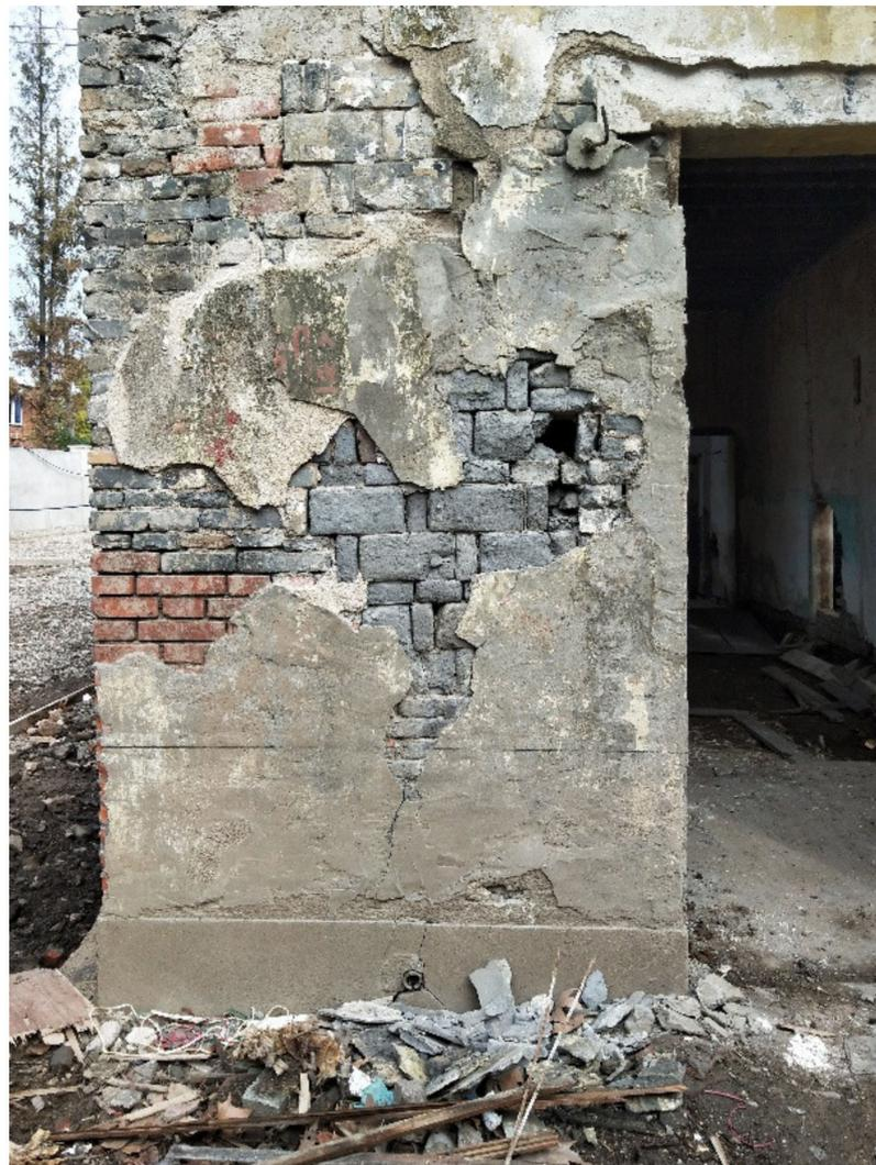
**Figure 21.** A wall made of different bricks of the “Tianbaoli” townhouses.
